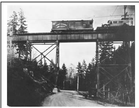
Steel High Bridge at Old Samish Road
